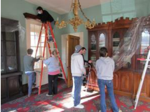
Wilson House staff and volunteers preparing for plaster repairs in 2013
