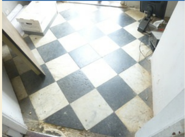
Tile flooring in the Court of Ordinary Building.
