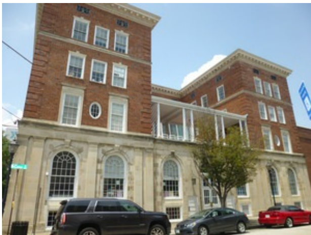
Former YMCA, undergoing rehab to accommodate TaxSlayer's downtown headquarters, 945 Broad Street.
