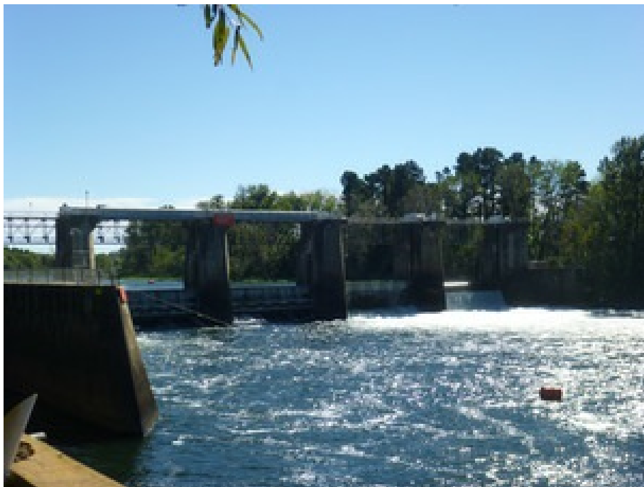
New Savannah Bluff Lock and Dam, listed on the 2018 Endangered Properties List
